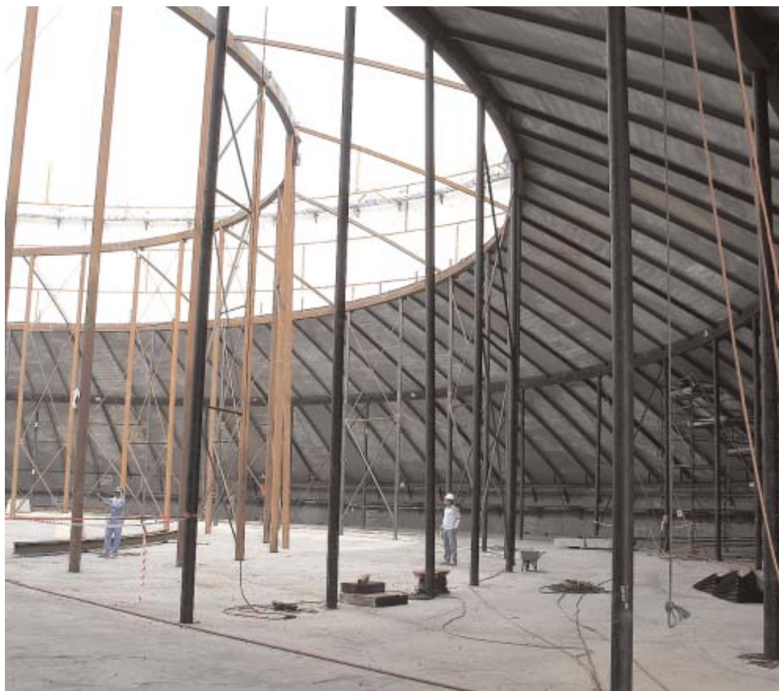
Equatorial Guinea LNG's tanks are now under construction for a 2007 start-up
